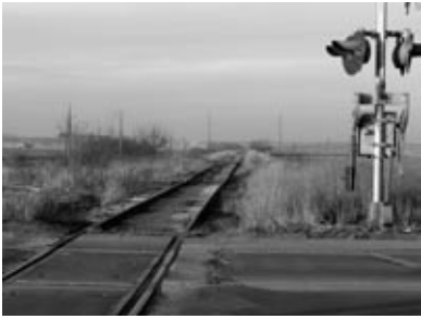
Fremont & Elkhorn Valley Railroad. A pioneering Rail-with-Trail project along this heritage passenger line will connect Fremont and Hooper.
